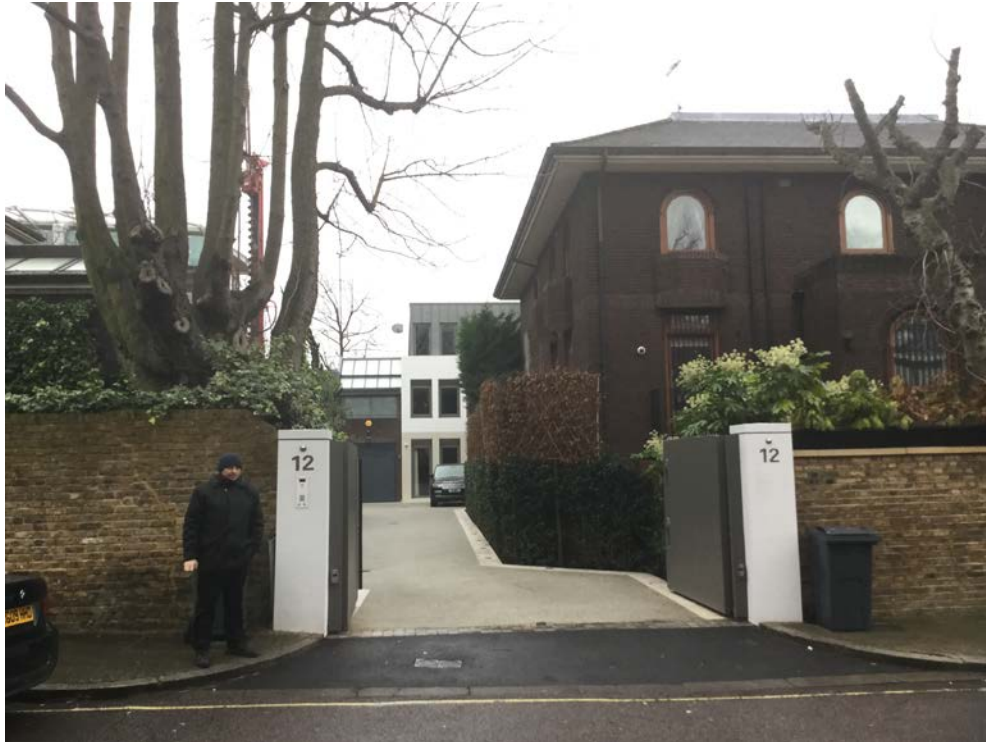
Shared Drive of 12 and 12A Elm Tree Road
